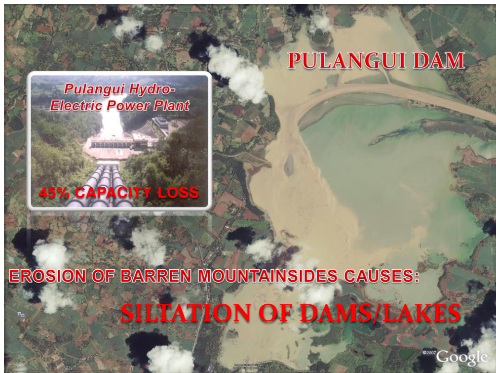
Figure 5. Siltation of Dam and Lakes
