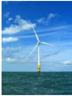
Vestas V90 Wind Turbine Kentish Flats
