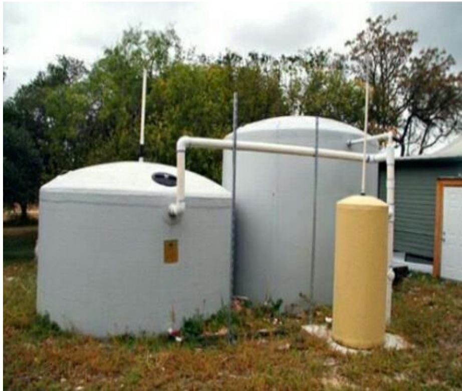
Fig 19: Rainwater Harvesting System
