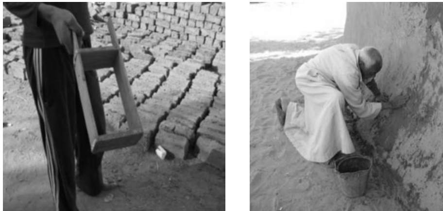
Photo 2.7: Traditional ways of building and craftsmanship in Omdurman using local materials that are about to vanish
