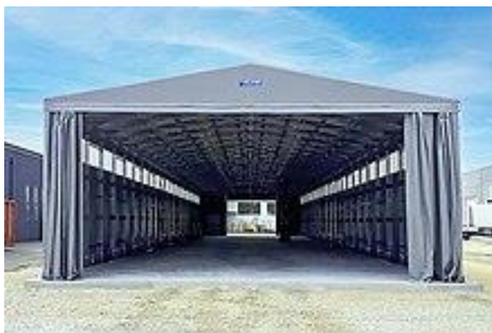
Tunnel Mobile in pvc
