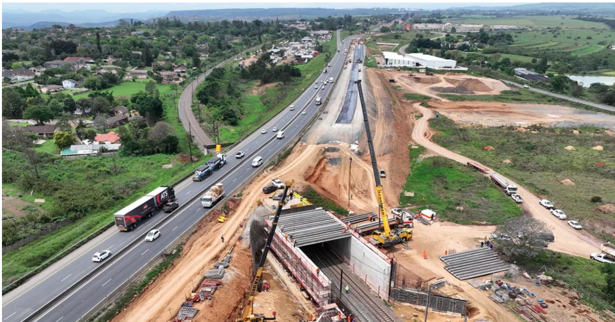
Figure 2 Infrastructure development Project under Construction in Uganda
