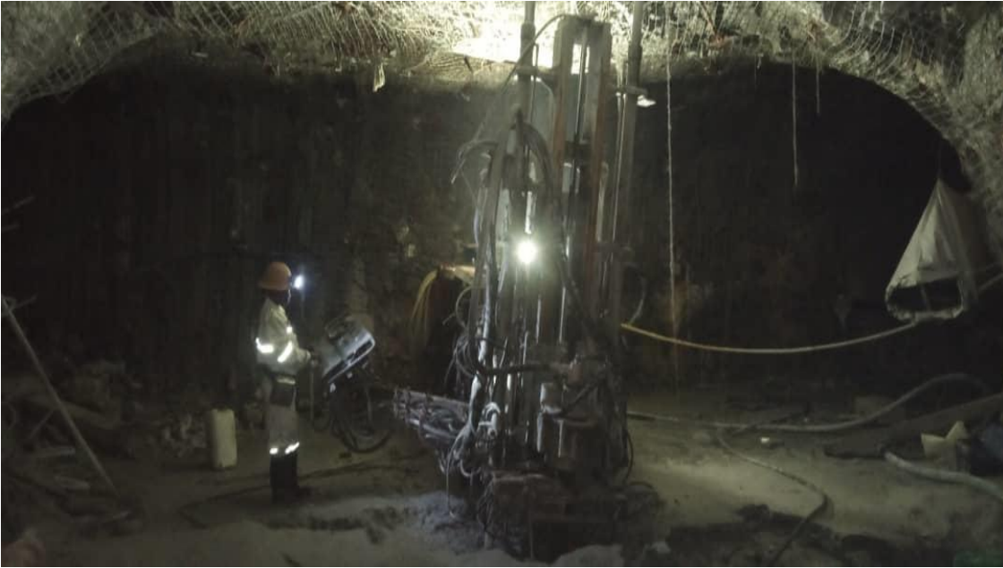
Figure 19: Cubex 16 drilling at 5570/280 VCR .
