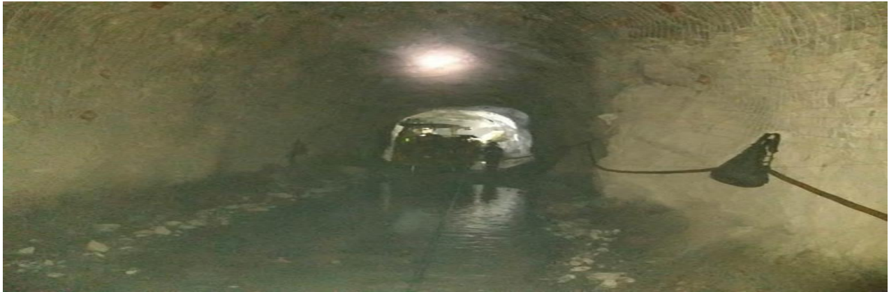
Figure 11: Depicting crosscut access to VCR chamber.
