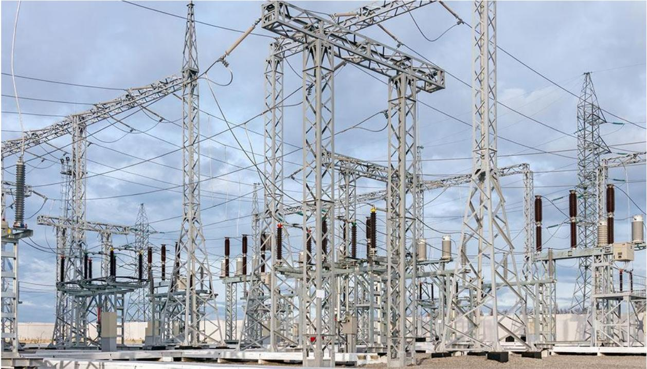
The collection MV/HV Substation collects the power from the PV plant/Wind farm. A ring system is utilized to maximize the number of PV/WTG IRR Units connected in series; however, radial systems are also employed in some PV/WF plants. MV power cables with cable terminations are utilized to connect medium voltage Ring Main Units (RMUs) in order to construct the MV PV/WF incoming feeder of the MV main switchgear.
