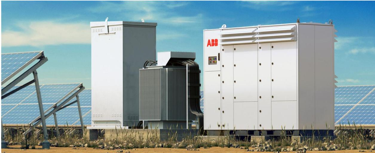
**Figure 2.1-14:** Central Inverter with Step-Up Transformer and RMU
