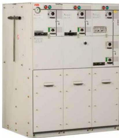
**Figure 2.1-22:** Ring Main Unit Three – Way
