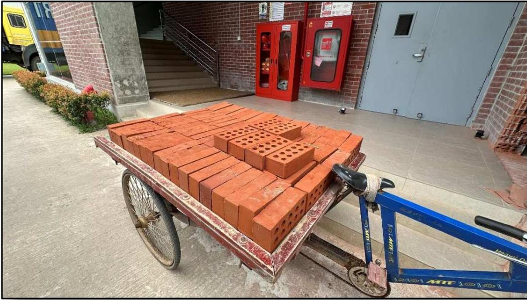
*Pic 5.4.13: 10-hole bricks used to build the walls of the building samples at site (Ref:ss)*
