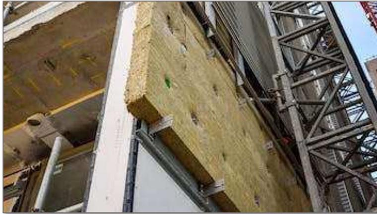
*Pic. 3.9: Rockwool insulation in walls and slab (Ref 3.10)*
